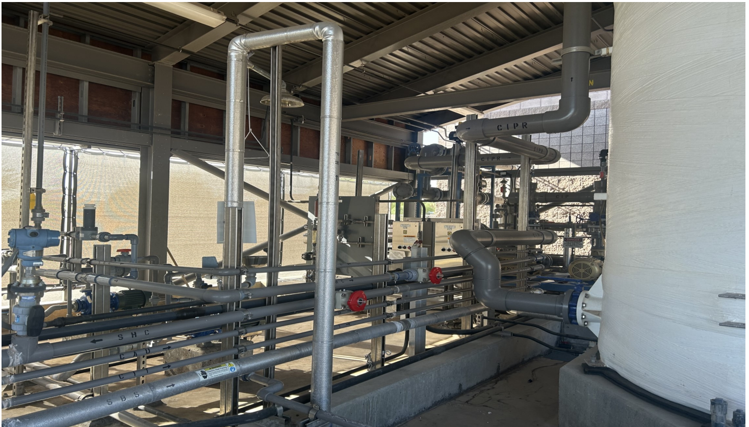
Bleach Piping Replacement Project Completed by Maintenance Staff
